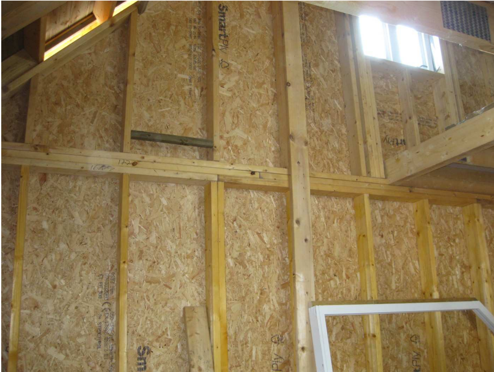
Gable Wall Adjacent to Staircase
