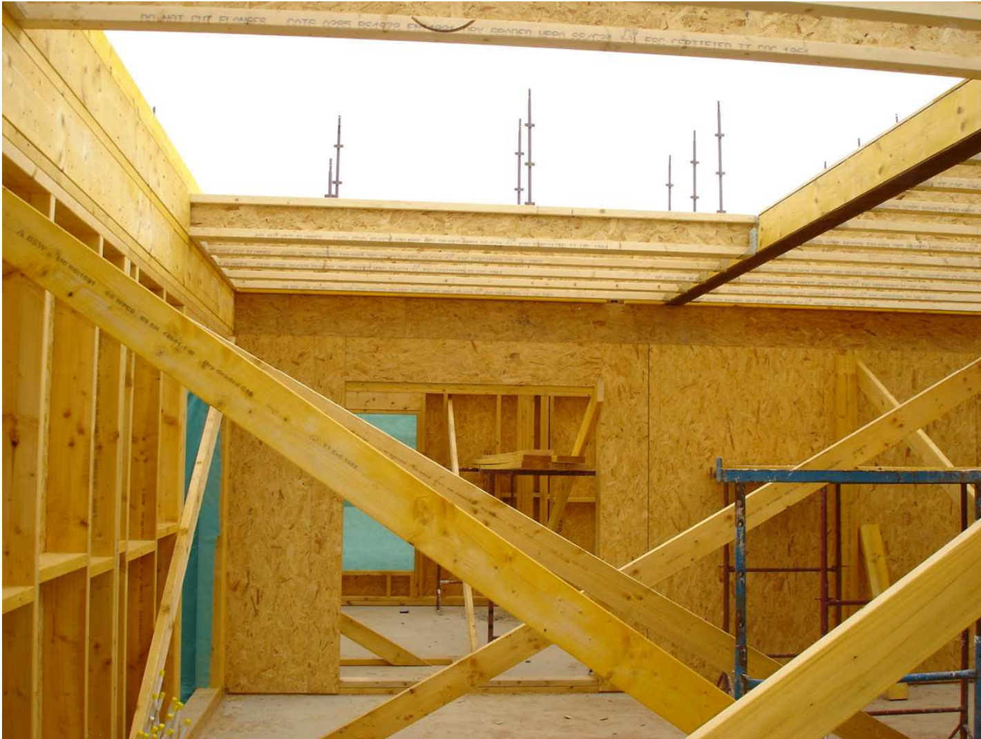
Timber Frame Construction with JJI Joist and Temporary Bracing
