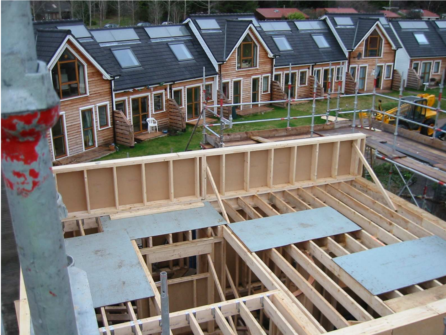
Solid Timber Floor Joists
