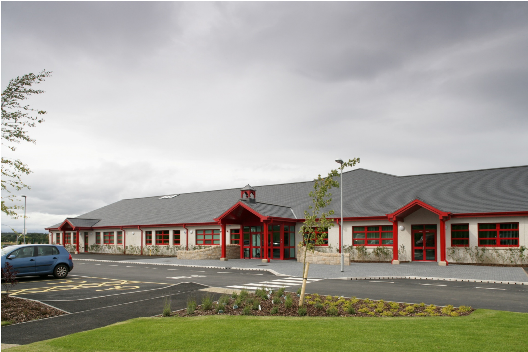
Block Clad Timber Frame Building
