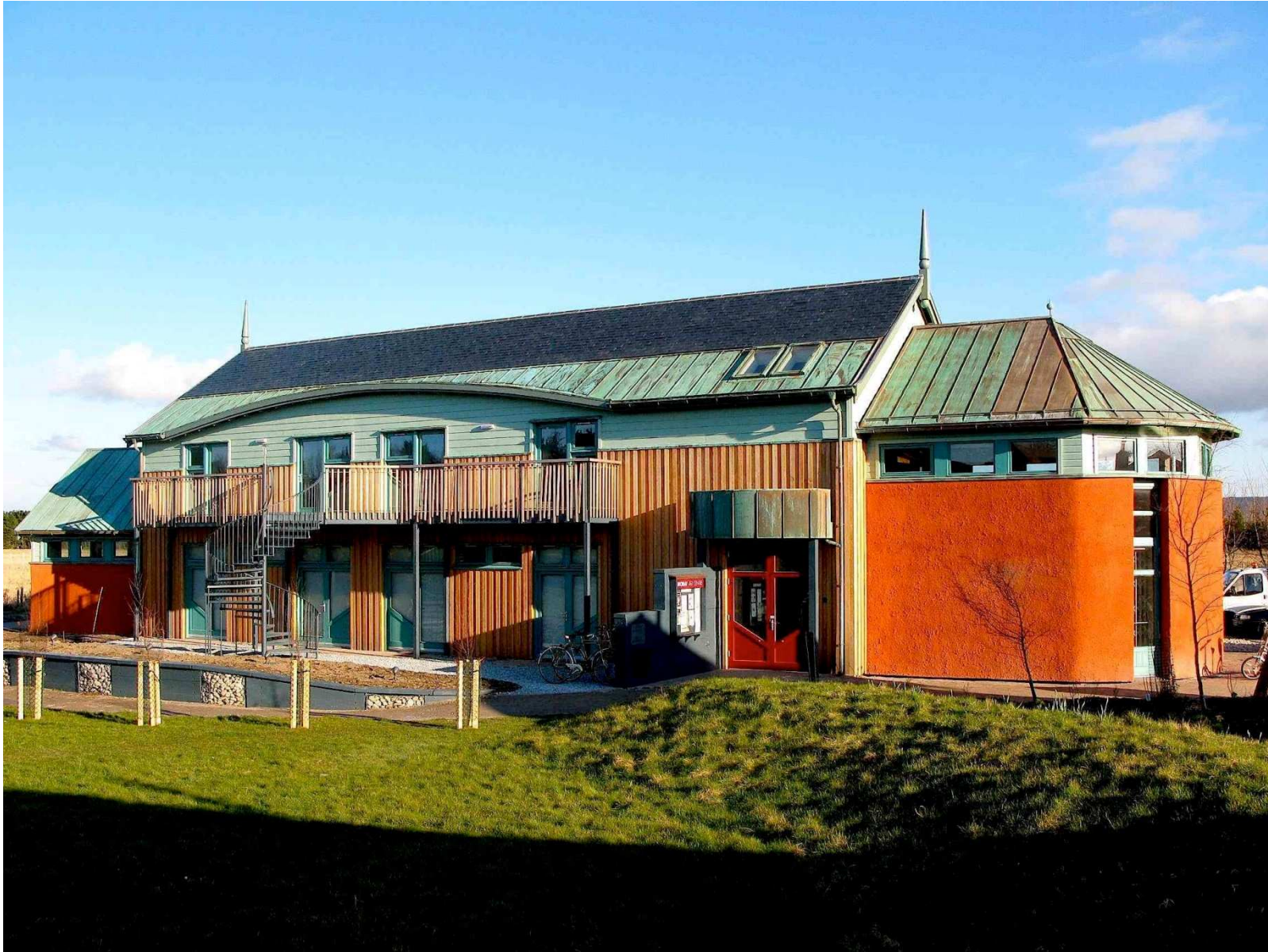
Timber Frame Building Clad in Various Materials
